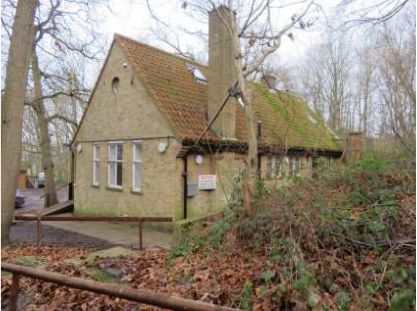
Entrance to Kelvedon Hatch – was disguised as large cottage. (Photo: Andrew Johnson – 2018)
