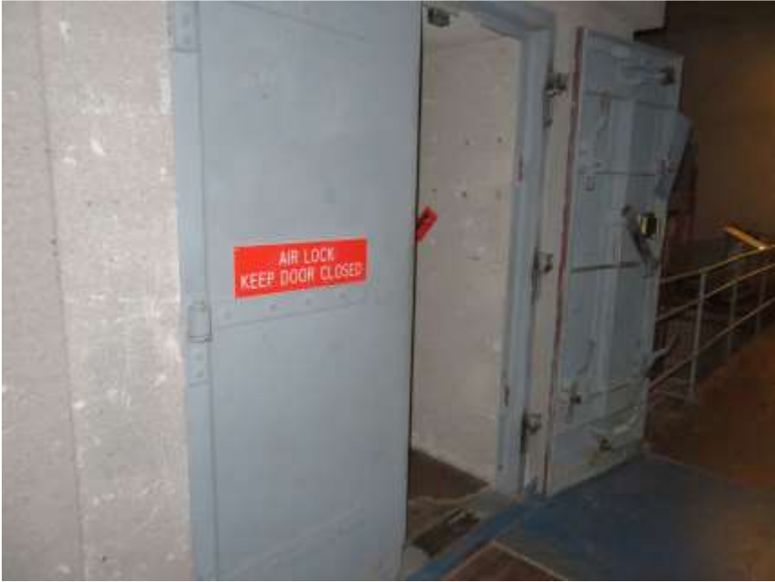
One of the doors which was meant to help keep out radiation/fallout following a nuclear attack. (Photo by Andrew Johnson – 2018)
